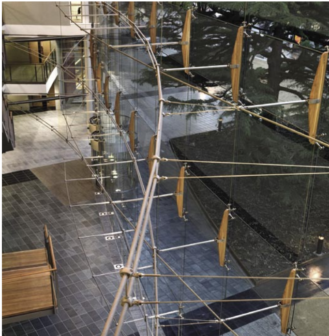
Fingal County Hall, 2002
