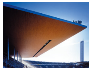
09_34_K2S Architects Ltd Olympiastadion Eastern Canopy 2005 Foto: Marko Huttunen
