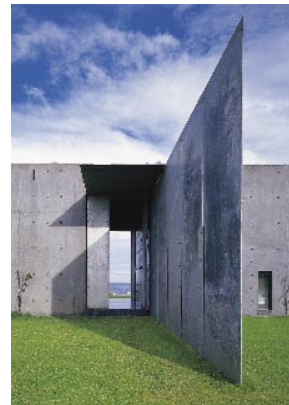
36a_DCM_Denton Corker Marshall Marshall House Phillip Island, Victoria, 1992 Entry from the courtyard Photo: John Gollings
