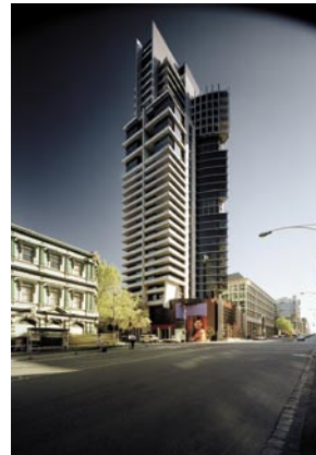
12_FKA_Fender Katsalidis Architects Republic Tower Melbourne, Victoria, 2000 Street view Photo: John Gollings
